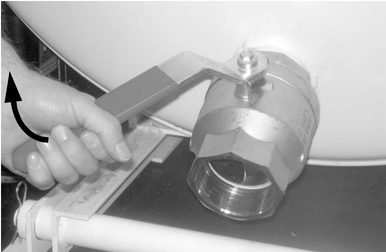
Figure 4-20. Close the tank drain valve when the liquid has finished draining.
