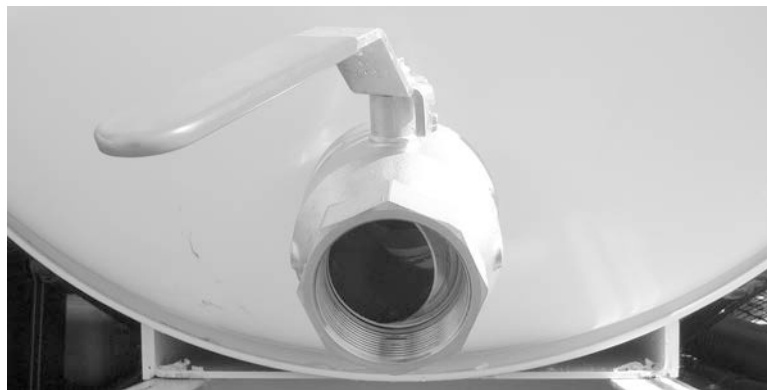
Figure 4-19. Check the drain valve before closing it to make sure there are no obstructions.
