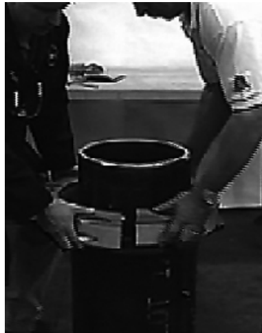
Figure 3-1. Attach the LCSF around the pipe as shown.
