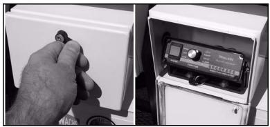
*Figure 4-12. Turn the lock counterclockwise to open the controller box.*
