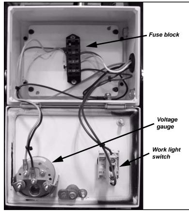
*Figure 5-4. Voltage meter and work light switch components and fuse block.*
